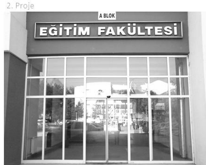
Figure 8. New entrance door of block A
