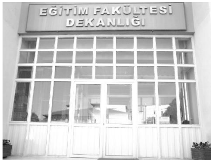
Figure 3. Entrance door of block A
